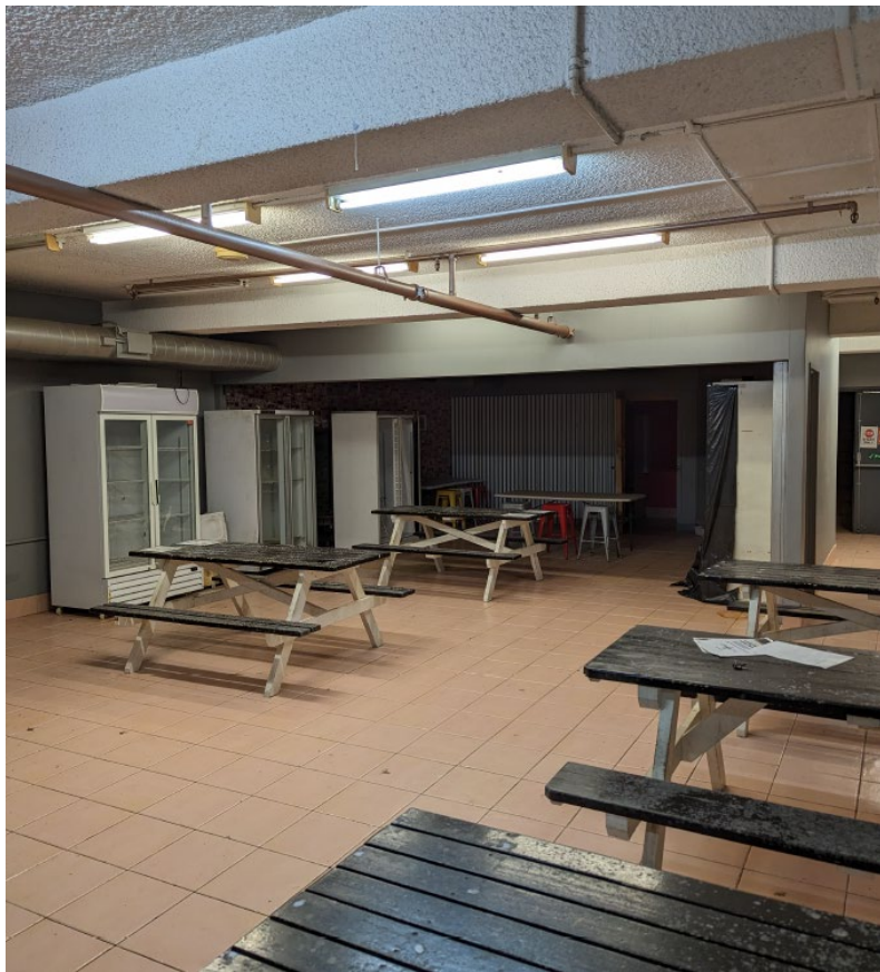
existing basement level 2
